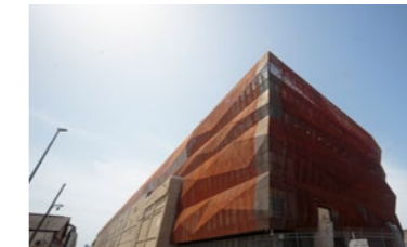
Interxion, MRS3, Marseille Data Halls: 6,900m 2 IT Power: 16.6MW
