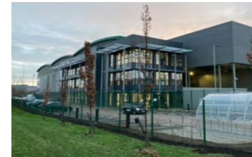
VIRTUS Stockley Park Campus, Stockley Park, London Data Halls: 37,000m 2 IT Power: 86MW
